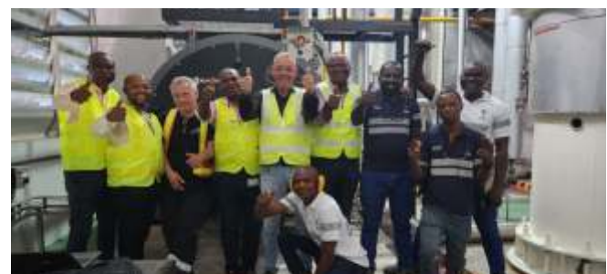
Successful installation of the first-ever dedicated biogas boiler in the HEINEKEN AME region at Ama Brewery, marking a significant milestone in our Net Zero journey.
