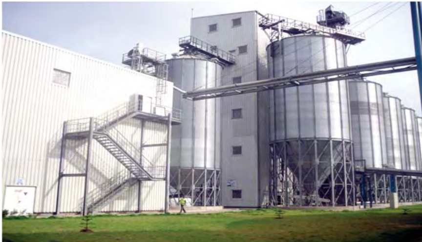
■ Steep House in Aba Malting Plant
