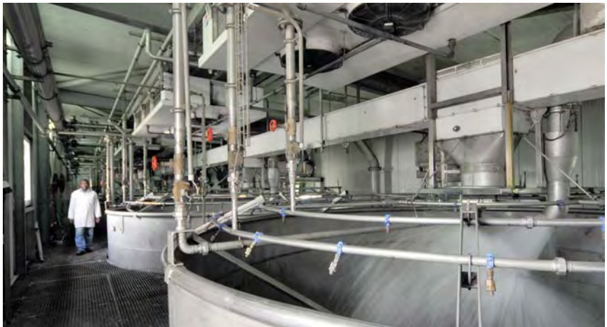
■ A section of Aba Malting Plant
