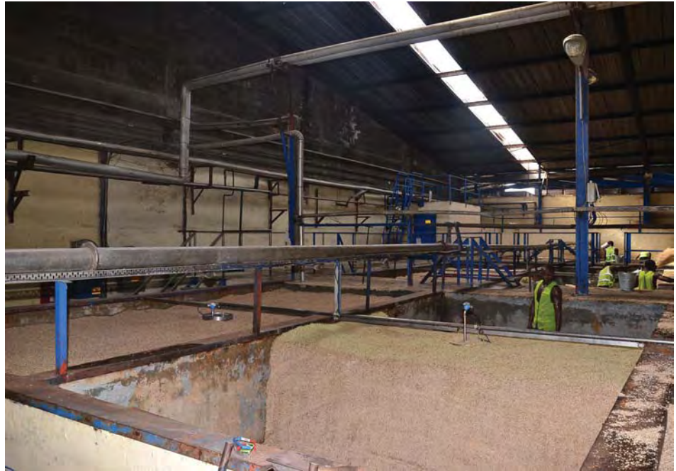
■ A section of Kudenda Malting Plant, Kaduna
