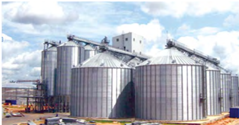
■ Raw sorghum storage silos
