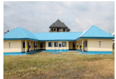
Newly constructed school block at Ngwa High School, Aba, Abia State.
