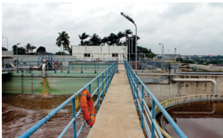
A section of Aba Wastewater Treatment Plant
