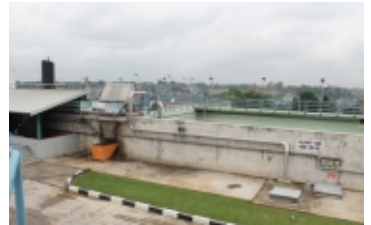
A section of Awo-Omamma Wastewater Treatment Plant
