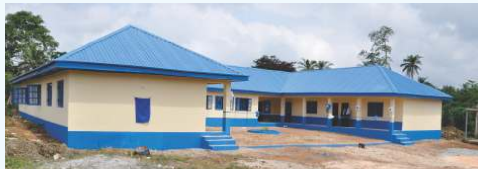
The block of classrooms donated by NB Plc to the school
